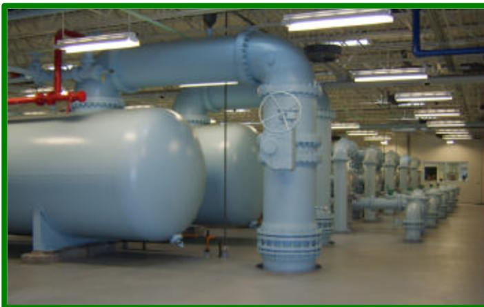
Two new Filtronics' *Electromedia*® I filters for iron and manganese were installed at each facility to add to the existing *Electromedia* filters put into service in 1991. Each of the filters is designed to run at 10 gallons per minute per square foot.
